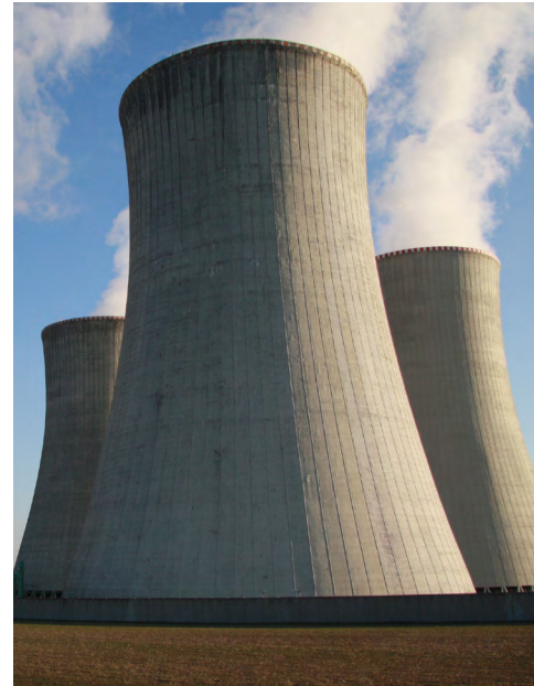
Figure 1. Cooling towers at a nuclear power plant
